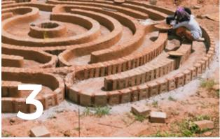
Shuttering to be done with plywood if pathway is straight or with brick if the pathway is curved.
