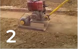
Subsurface should be compacted well with earth rammer machine/road roller. Compaction area should be done with minimum 1 feet buffer on both sides of pathway.
