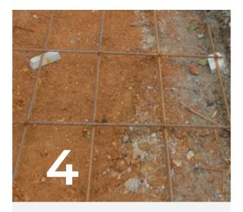
Steel reinforcement for the grade slab - 8mm Diameter TMT road @ 300mm C/C Spacing should be laid on both directions with 1" bottom covering.
