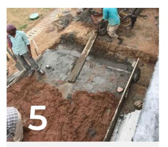
A normal concrete (3") is laid out in the given proportion. With an additional mix of 2 bags of red soil to the concrete mixture, the mud concrete is poured to form 3" thickness.
